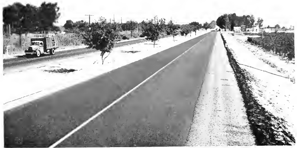
Divided sector of U. S. 99 between Selma and Fowler. New south-bound traffic lane on right. Old highway on left
